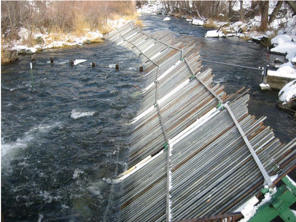
Figure 1. Alaska-style panels of the Shasta River Fish Counting Facility.
